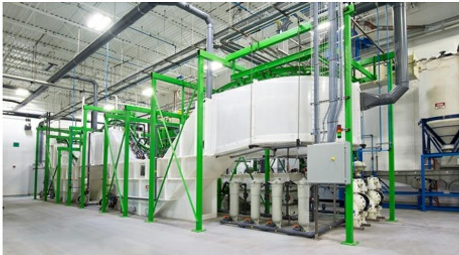
A recycling facility gives photovoltaic panel producer First Solar a way to extract components from defunct solar panels for eventual reuse. Photo courtesy of First Solar
